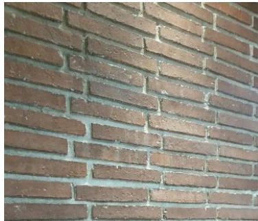
Figure 1: Example of Klompie brick detailing
